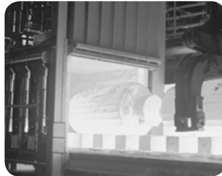
Bogie hearth forging furnace in the metallurgical industry
